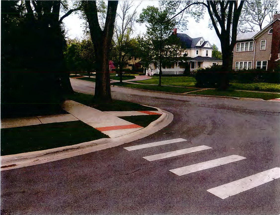
VIEW OF OBSTRUCTION ON SOUTHEAST CORNER (APRIL 2017 – westbound Walnut looking southbound on Garfield)
