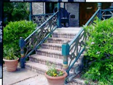
Compatible additions and replacements - Front railings hand made to match original. Side porch in addition (above) matches original and incorporates posts from original rear porch.
