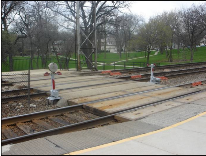
Figure 6.7: Existing Highlands Metra Station Crossing
