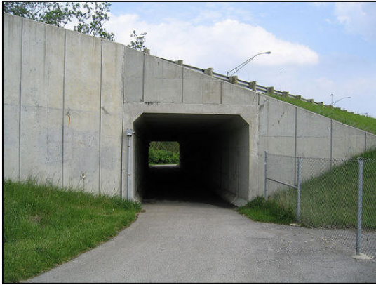
Figure 6.9: Typical Box Culvert Tunnel (Source: www.flickr.com )
