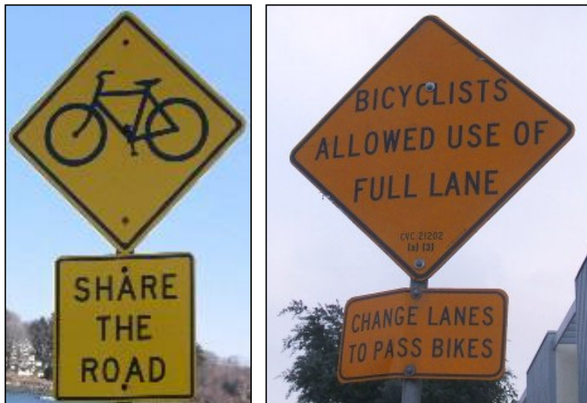
Figure 6.12: Two examples of regulatory signs for shared lane bike facilities (Source: Dolben.org)
